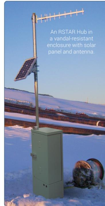
An RSTAR Hub in a vandal-resistant enclosure with solar panel and antenna.
